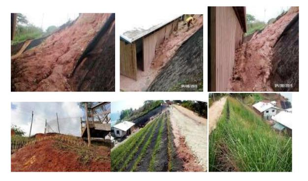
Extensive erosion and land slips on unprotected slope causing severe damage to buildings prompted authority to adopt Vetiver System Technology
